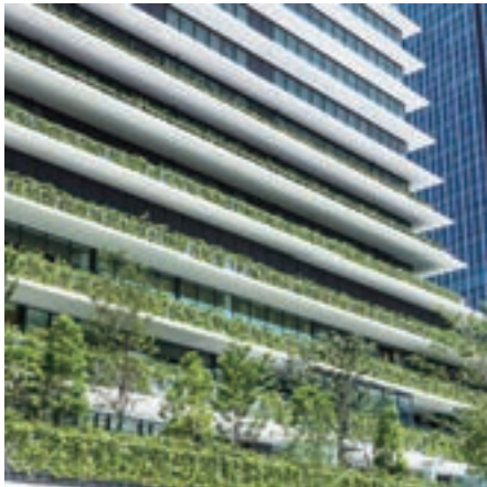
Eaves of building exterior walls that block direct sunlight
